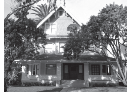
Jim and Janice Robinson's restoration of the Victorian era Teed Residence in University Park has won an HPOZ Award. Along with exterior repainting, the work involved the reproduction of 50 rafter tails and scrolled bargeboards
