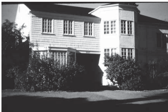
The John L. Matheson/Church of Jesus Christ of Latter-day Saints Residence in a 1941 photograph, while it was serving as the California Mission headquarters for the Mormon Church.
